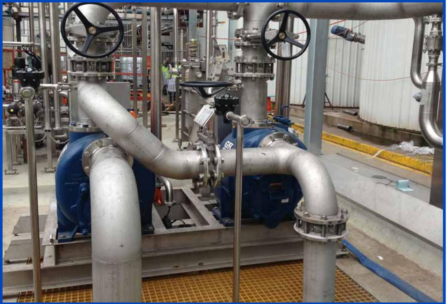
Gorman-Rupp Pumps are mounted “high and dry” above the wastewater for safe and easy access for monitoring and service
